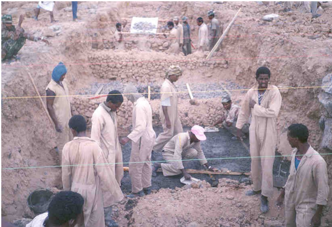
Figure 2 Lean concreting at Assab construction site.
