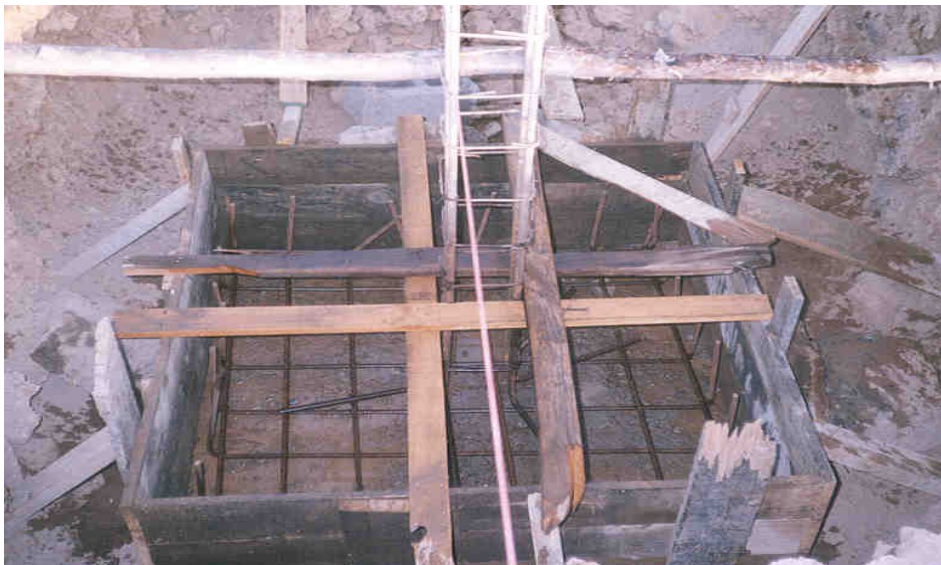
Figure 4 Single spread foot foundation utilized at Assab hospital.
