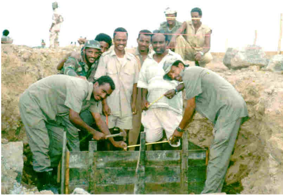
Figure 5 Foundation formwork placement.
