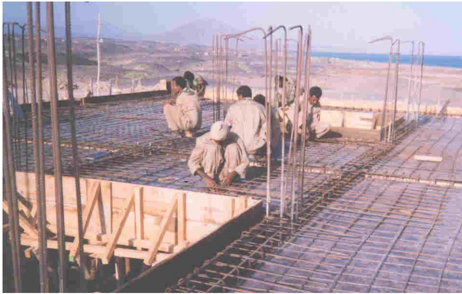
Figure 9 First floor reinforcement placement.
