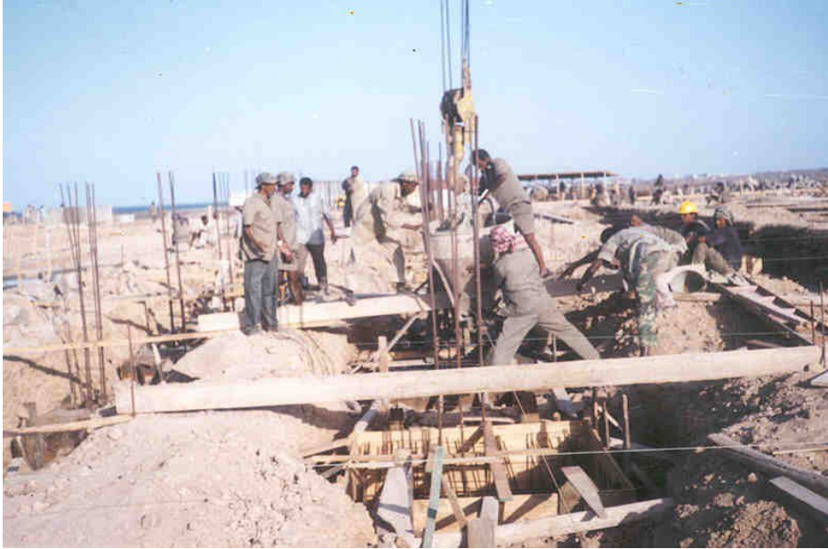
Figure 3 Constructing the foundation and columns of Assab referral hospital.
